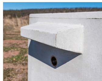
Reinforced Concrete Hob
