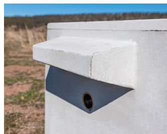
Reinforced Concrete Hob
