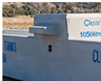
Reinforced Concrete Hob
